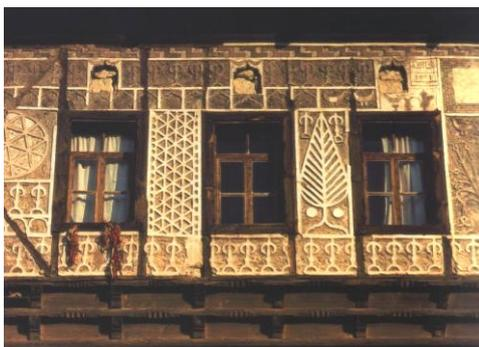
**Figure 12. Application of Malakari technique on the façade of room - Mektepçiler House. [3]**
