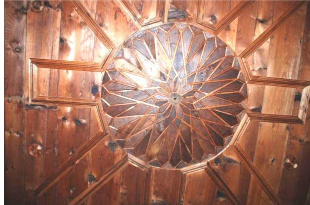
**Figure 6. Ceiling and lath-and-plaster workmanship with Citakari technique - Kileciler House.**
