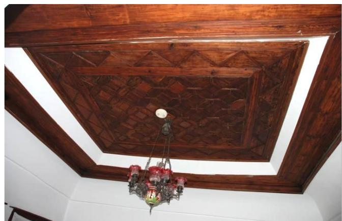
**Figure 11. Lath-and-plaster workmanship of the ceiling representing Cítakari artisanship and its joint with the wall - Kaymakamlar House.**
