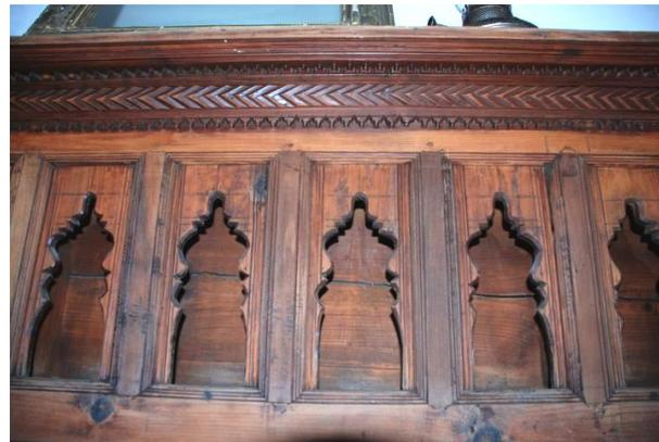
**Figure 8. Niches constructed via saw carving and chipping technique - Kaymakamlar House.**
